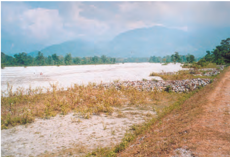
Photo 34. Dry active left channel of Pana river with embankment protecting Chuapara Tea Estate, November 2005 (by L. Starkel)
