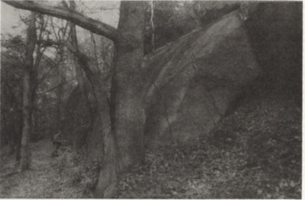
Photo 2. Sheeting planes on the western slope of the Witosza hill
