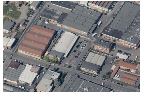
Figure 2. View of a small area inside Villaggio Artigiano , where the specific mitigation measures were applied, in particular to the car park, which is clearly visible in the center of the selected area
