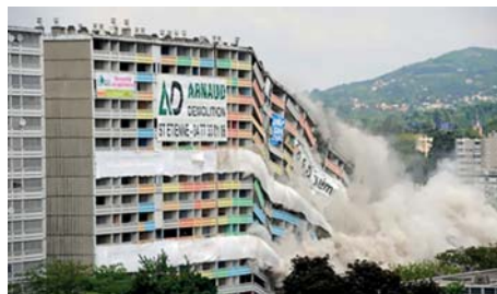
Figure 1. Explosive demolition of a slab of approximately 300 housing units
