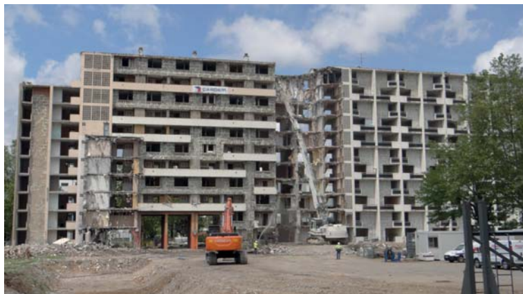
Figure 2. Demolition by nibbling of a slab in Mermoz, Lyon (2013)
