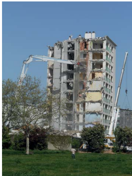
Figure 4. Demolition by nibbling of a tower in Bron-Terrailon, Bron (2013)
