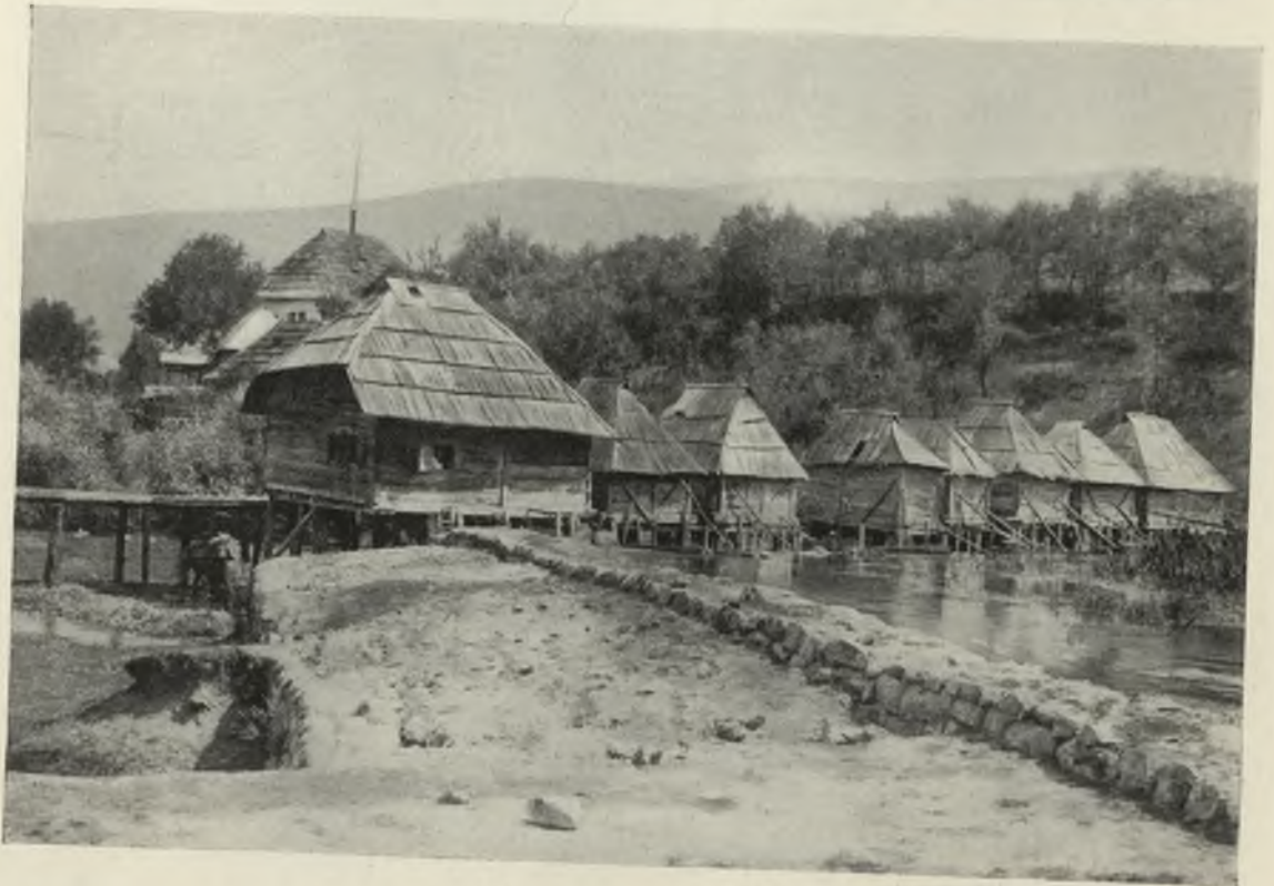
507 MILL HOUSES AT ILIDŽE
