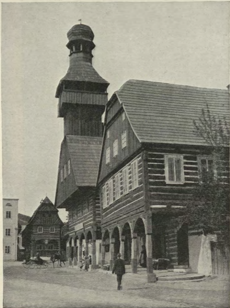
252 OLD "RATHHAUS" AT EISENBROD, NOW DEMOLISHED
