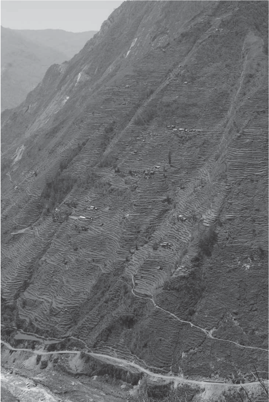
Figure 6. Terraced fields on a steep debris slope, middle Kali Gandaki valley (1,200 m, Myagdi District). The new road is cut into the instable foot slope. (© M. Fort, 2009)
