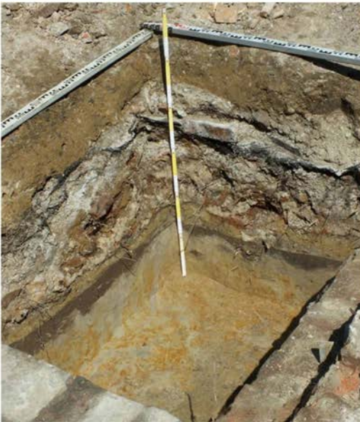
Fig. 5. Remains of a preserved insulating layer under the floor in the form of a sheet of tar paper: 1– Birkenau, barrack B-167; 2 – Jawischowitz, block no. 6. Photo: K. Peschel and W. Tabaszewski.
