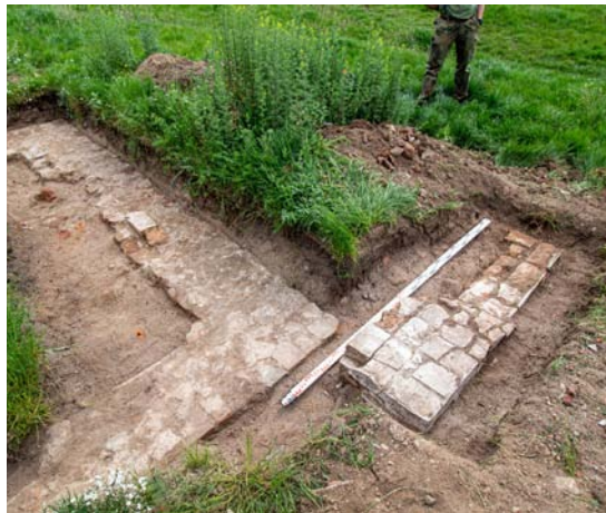
Fig. 13. Kutno. The foundation at the southwest corner of the ohel , view from the northwest. Photo: J. Ginter.
