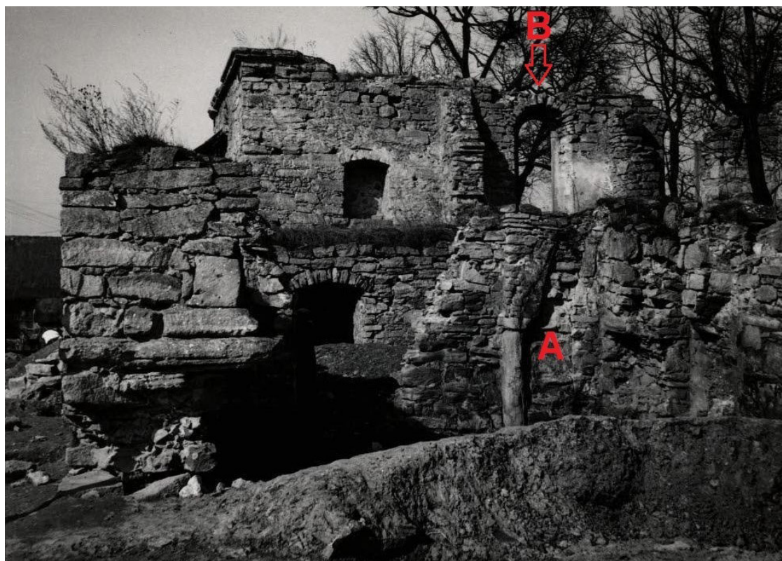
Fig. 15. Complex of the Holy Spirit in Szydłów, view from the south. In the foreground south hospital wing, hospital church in the background: A – The pillar and smoke duct of the hearth (Three and Four Phases); B – The finial of the hospital church window, ca. 1970. Photo: Author unknown, Collections of the Szydłów City Hall.
