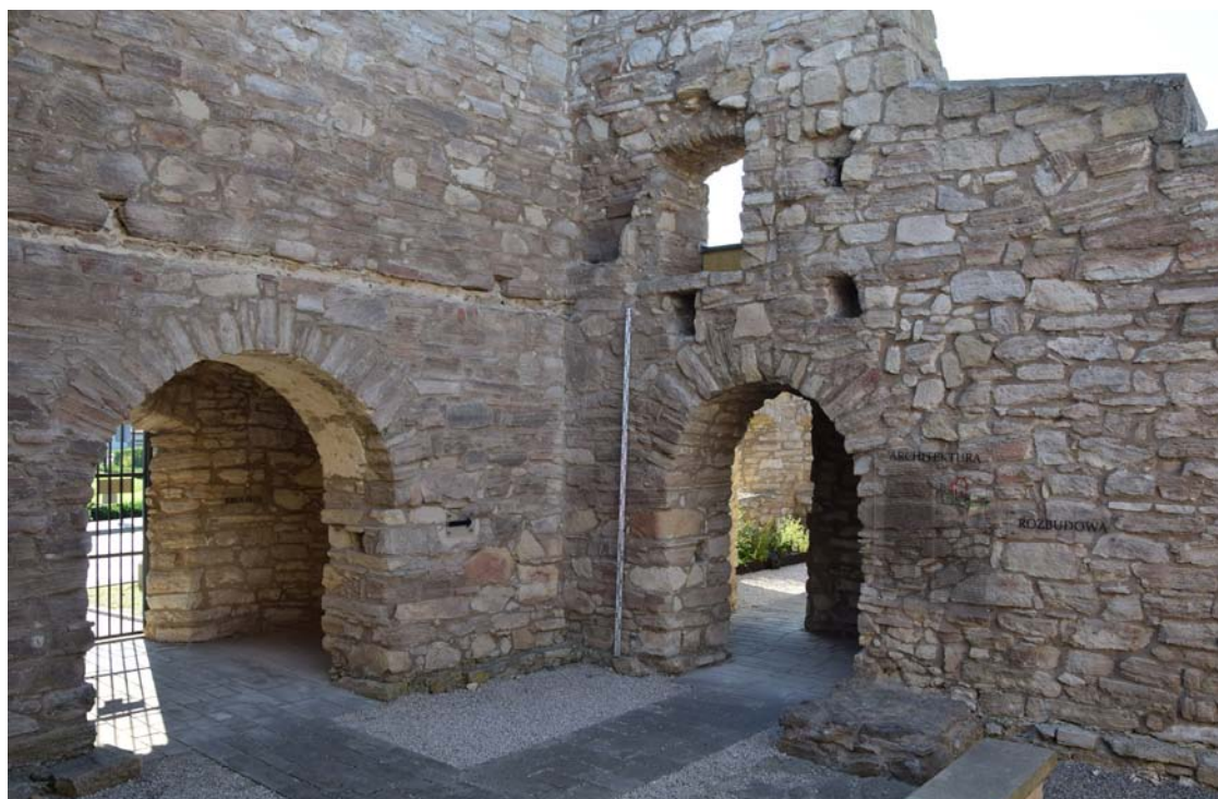
Fig. 11. Complex of the Holy Spirit in Szydłów, the nave of the hospital church: view towards the southwest, on the left side the western corridor and on the right side north corridor of the ambulatory porch. On the right side in the background Patients' room in the north hospital wing. Condition after conservation, 2025. Photo: T. Olszacki.
