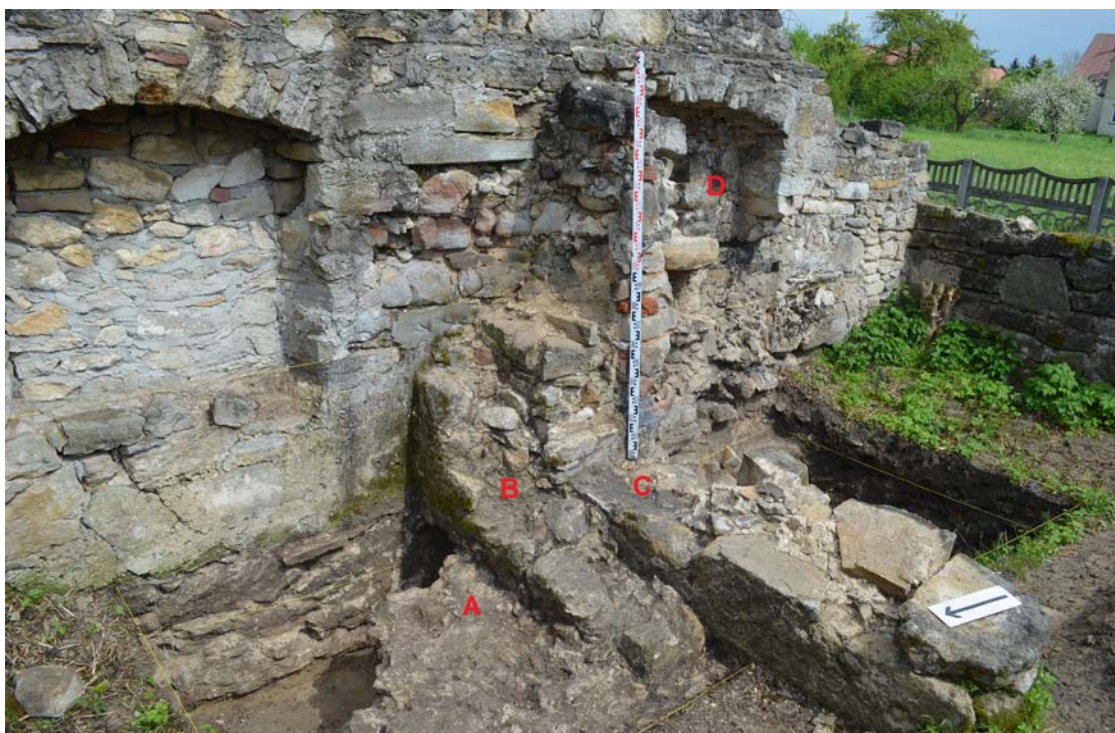
Fig. 14. Complex of the Holy Spirit in Szydłów, the south hospital wing, the archaeological trenches 2 and 9/2017: A – Hearth inside the Phase Two hospital; B – Fireplace inside the hospital of Phases Three and Four; C – Shaft between hearth and fireplace of Phases Three and Four; D – Small window-vent in the hospital's east wall of the Phase Two, later bricked up, 2017. Photo: T. Olszacki.
