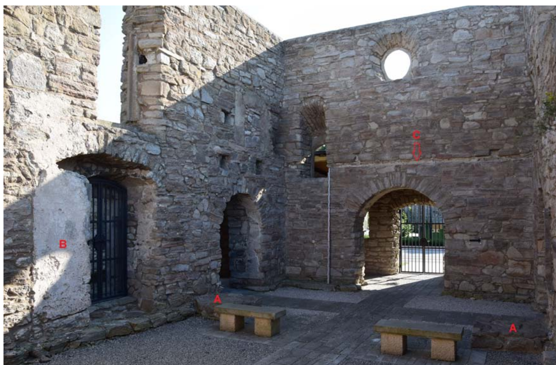
Fig. 10. Complex of the Holy Spirit in Szydłów, the nave of the hospital church: view towards the southwest with the western corridor of the ambulatory porch visible in the background: A – fragments of the western wall of the church of the Phase Two; B – partial bricking up of the panel niche of the Phase Two, and carving out a door opening in it in the Phase Three; C – former floor level of the gallery. Condition after conservation, 2025. Photo: T. Olszacki.
