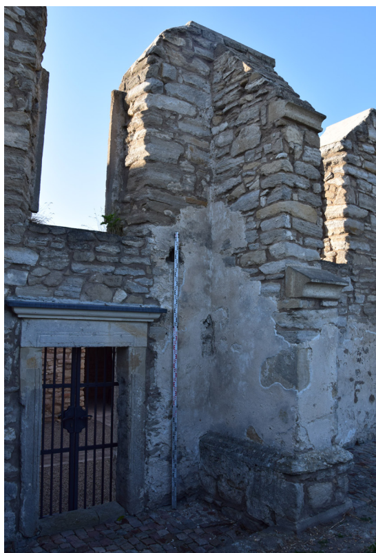
Fig. 9. Complex of the Holy Spirit in Szydłów, view of the hospital church from the south: side portal and buttress of the Phase Three. Condition after conservation, 2025. Photo: T. Olszacki.
