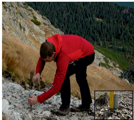
Figure 3. Installing a benchmark
