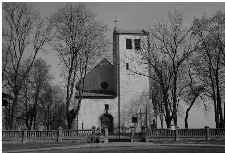
Fig. 3. Structures built of calcareous marl. Sobótka, Poddębice district (a), Wilamów, Poddębice district (b). Photo: I. Sobkowiak-Tabaka.
