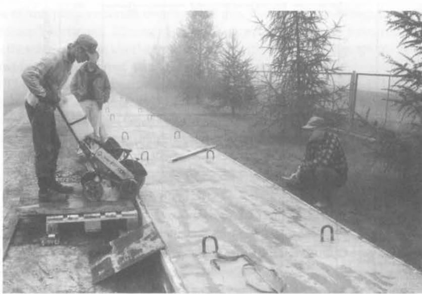
FIGURE 20. Zmigrod tests: notching the overlaid slabs.
