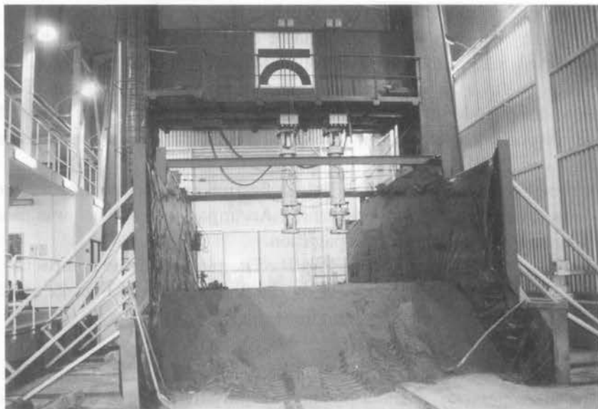
FIGURE 22. Placement of the soil, compacted layer after layer.
