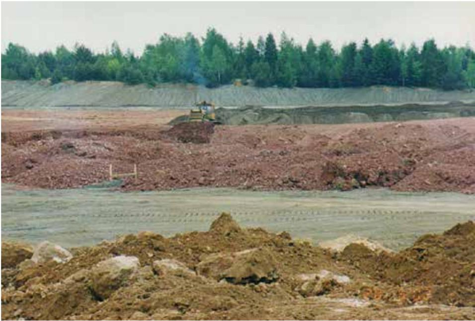
Fig. 15. Reclamation of an open-pit performed by backfilling with flotation tailings, 2002 (photo B. Włodarz)
