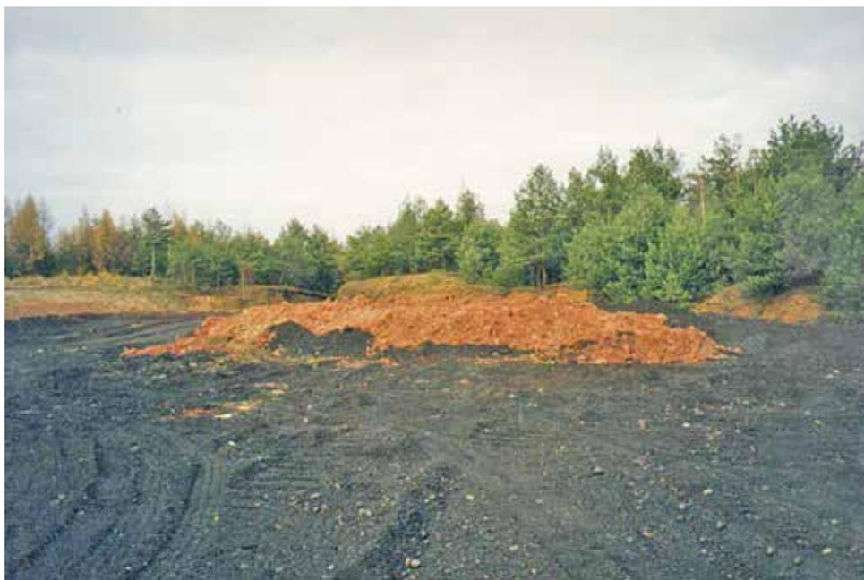
Fig. 14. Reclamation of an open-pit performed by backfilling with slags, 2002 (photo B. Włodarz)
