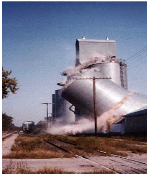
Figure A.3. Collapse of a granular (corn) silo due to a poor design.
