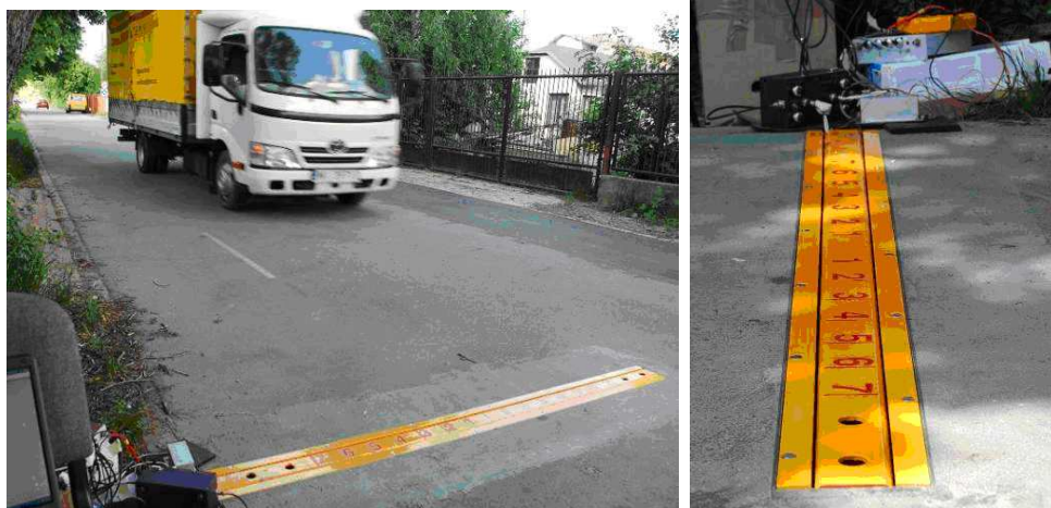
Figure 2.23. Second version of the beam-shape WIM device mounted on public road.
